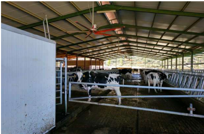
CENTRAL LECHERA: INTERIOR NAVES
